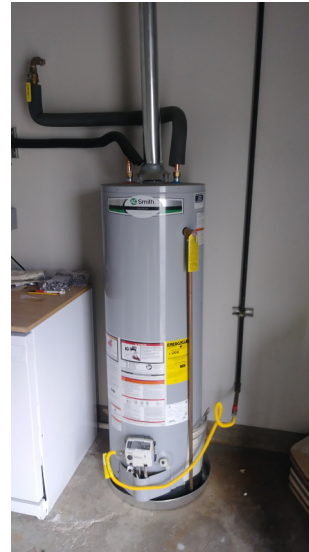
STORAGE ROOM/KILN ROOM- DEMO (E) WATER HEATER
